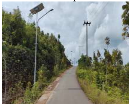
Figure 9. There is Street Lighting but Inadequate for Community Activities at Night
