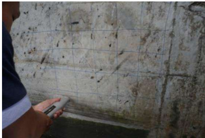
Gambar 16. Pengujian Hammer Test di Spot Spillway Inlet – Spot 1
