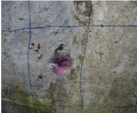
Gambar 6. Pengujian Karbonasi di Spot Spillway Inlet – Spot 1
