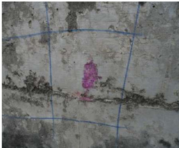
Gambar 7. Pengujian Karbonasi di Spot Spillway Inlet – Spot 2
