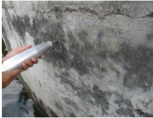
Gambar 5. Pengujian Hammer Test di Spot Spillway Inlet – Spot 2
