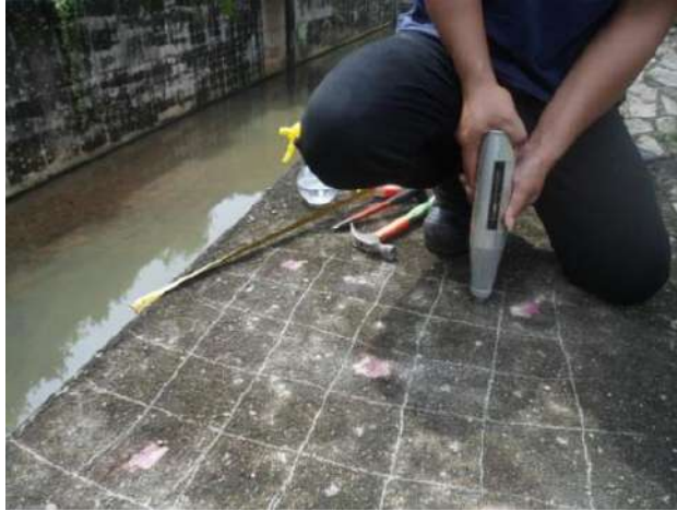
Gambar 19. Pengujian Hammer Test di Bottom Outlet – Spot 1
